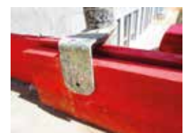
Fig. 18 Support de plinthes
